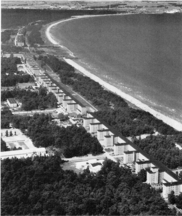
Aerial view of the Prora complex looking north
